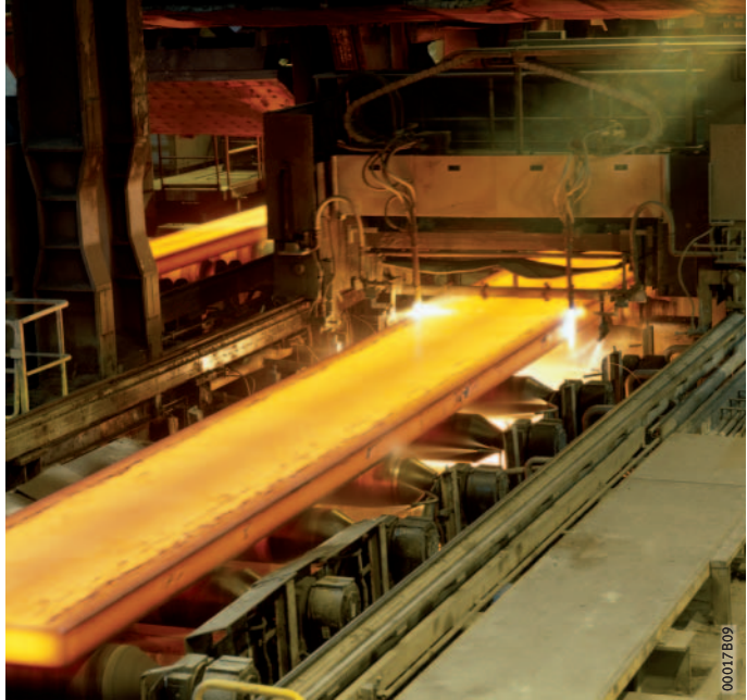
Figure 1 Continuous casting plant
